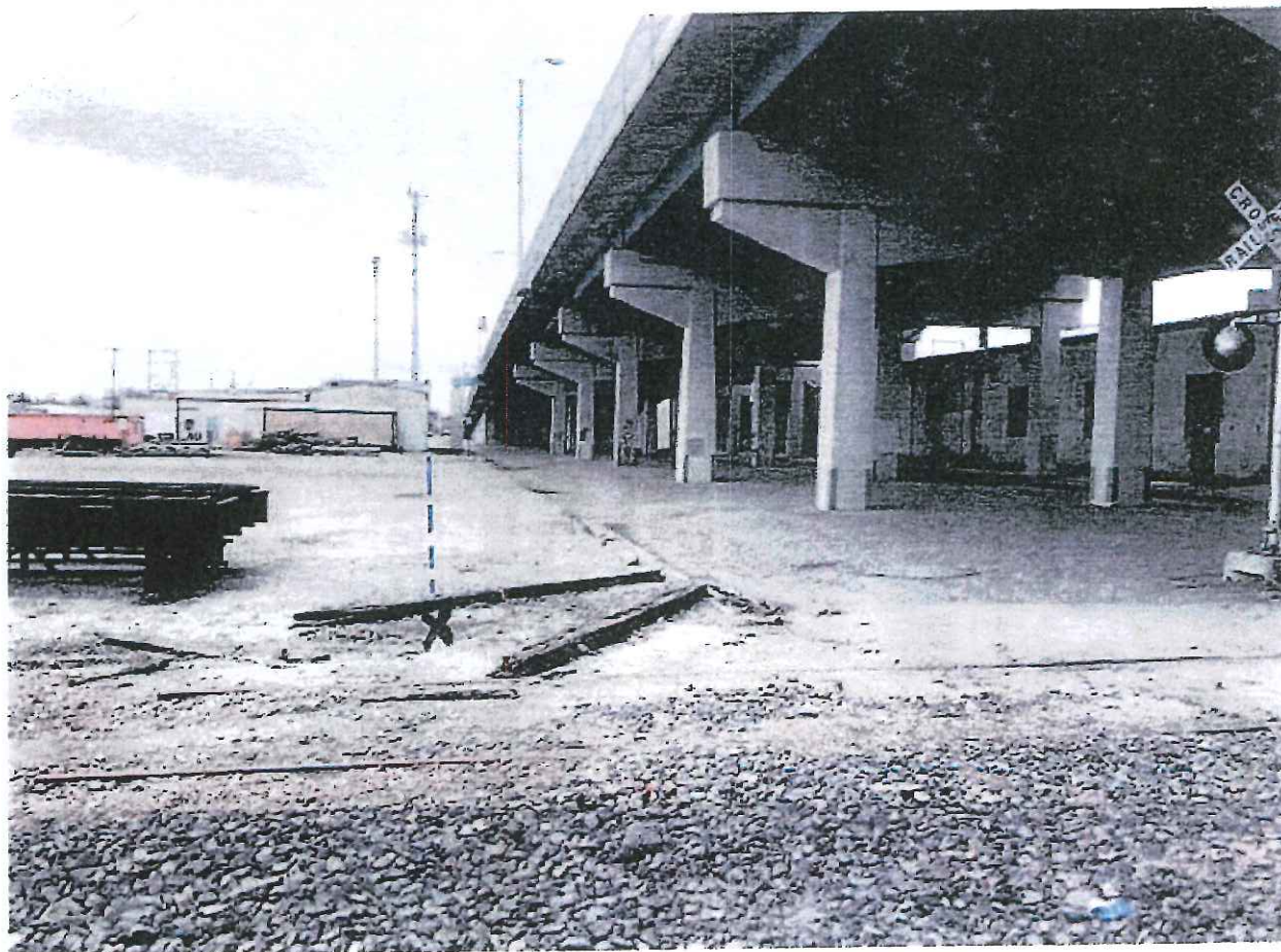
LOOKING NORTH ALONG BOTTLING EAST
