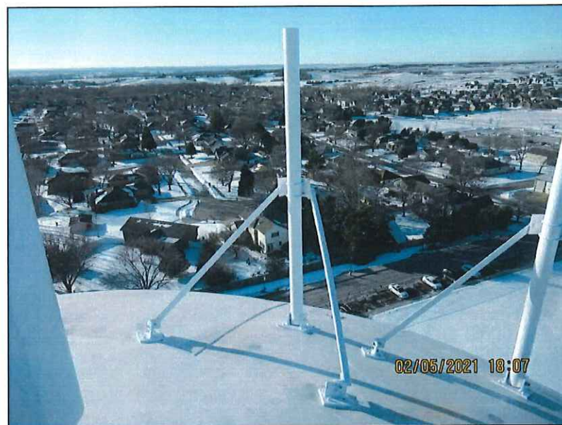
New antenna mounts on top of water tank
