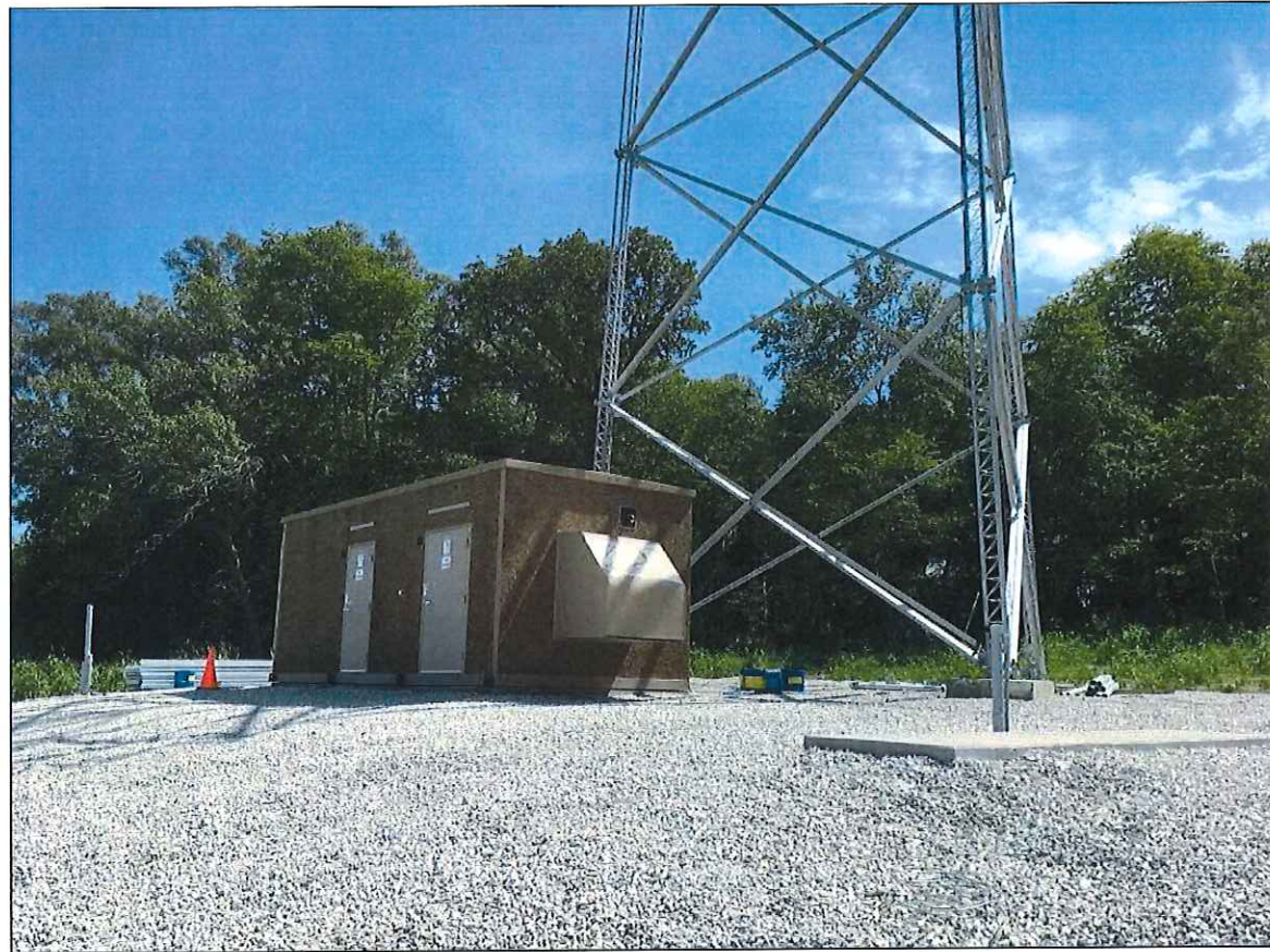
Hooper Shelter and Tower (prior to fence installation)
