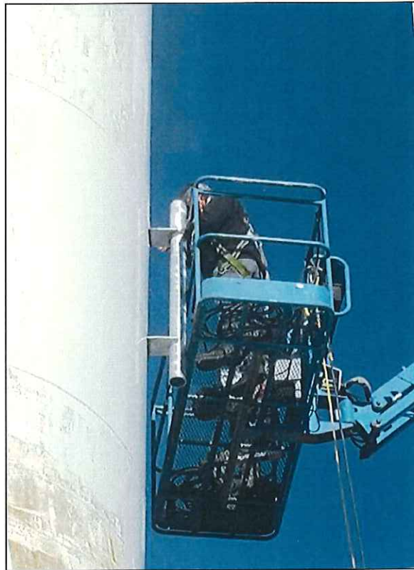
Welding antenna mount on side of tank structure
