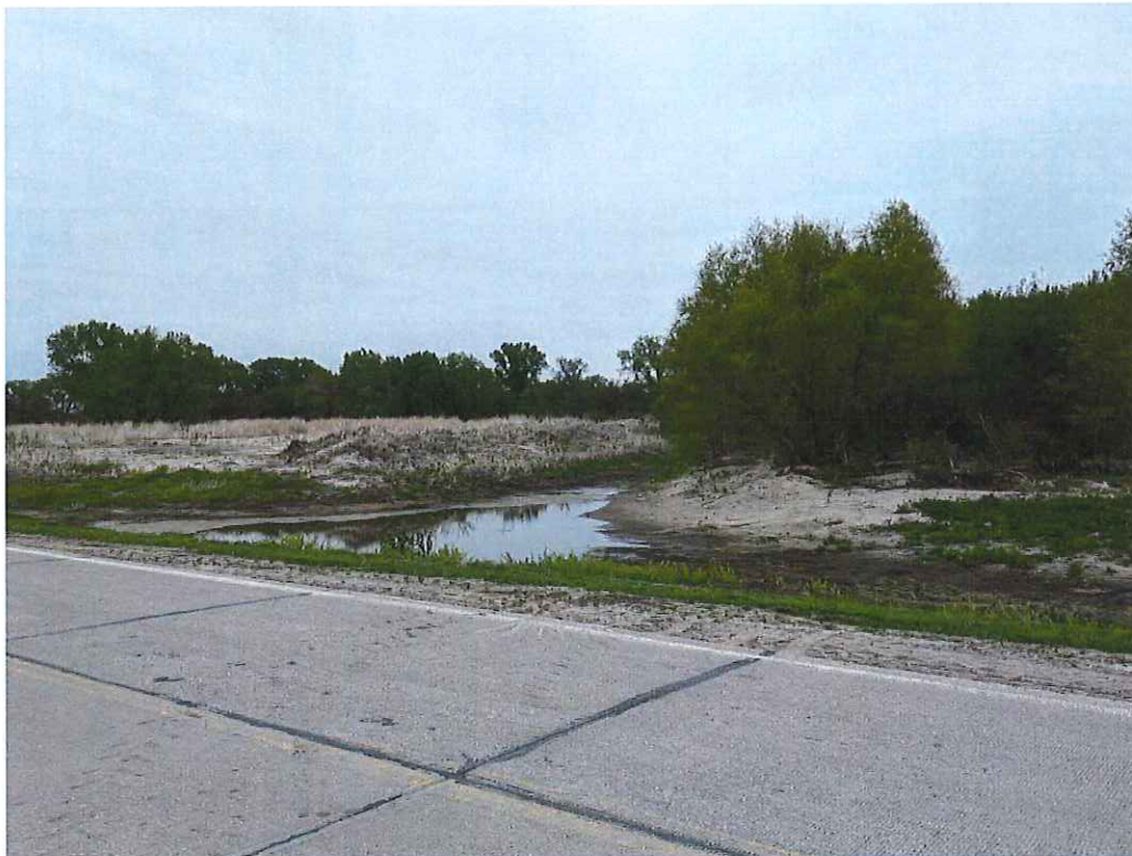
Picture 6: Dike 3: looking at South side of culvert toward "flood channel"
