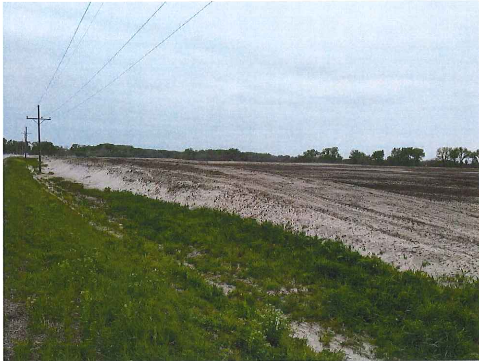
Picture 3: Dike 2, general view looking from East to West
