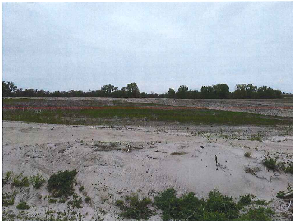
Picture 4: Dike 3, general view. Note: curvature of dike
