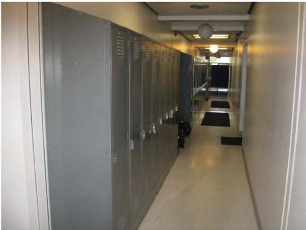
Corridor Link between FPD offices and garage, with officer lockers
