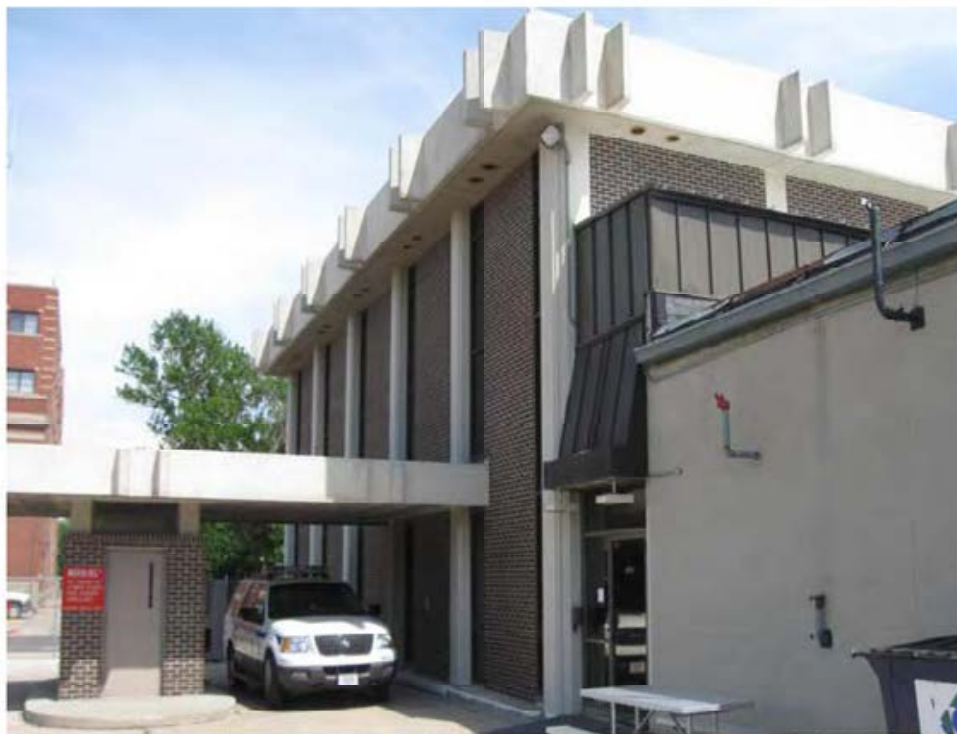
Former teller kiosk/canopy, plus reroofed standing seam roof over corridor link to garage
