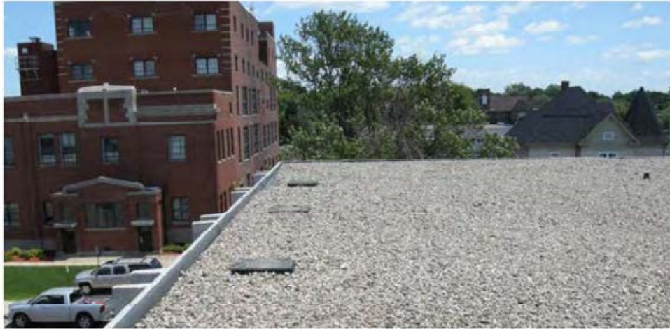
Roof column caps for potential future Third Floor.
