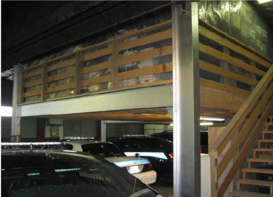
Evidence Storage mezzanine in garage
