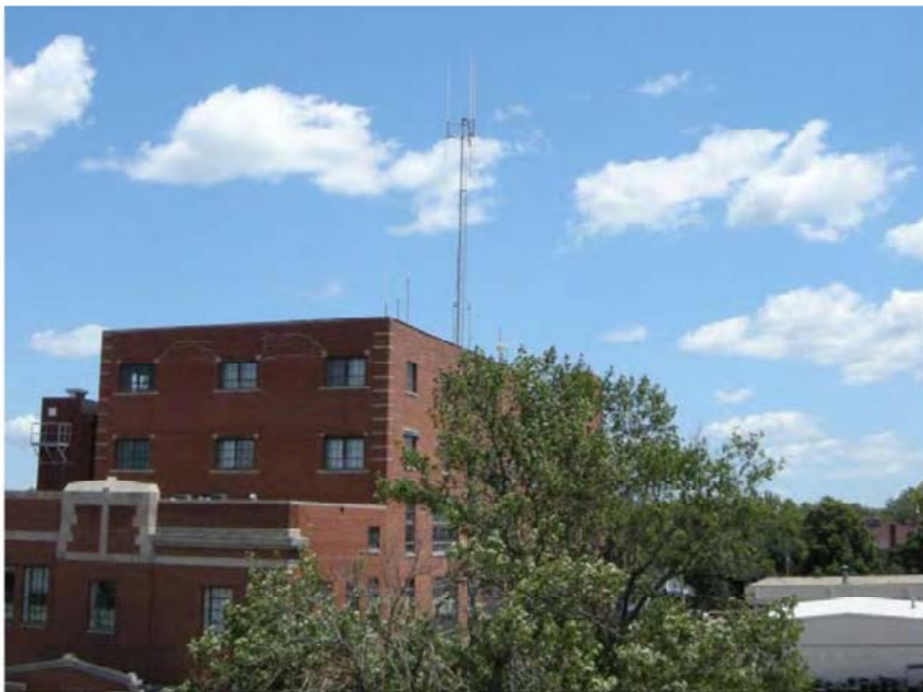
Dispatch tower on Power House apartment building
