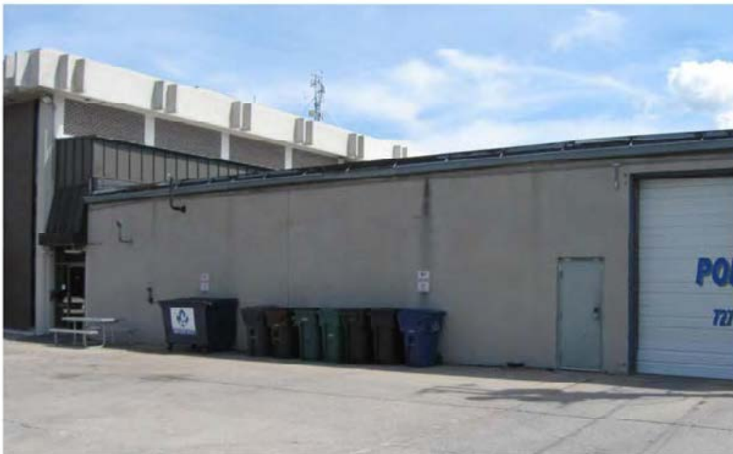
Unenclosed dumpster and trash receptacles behind garage
