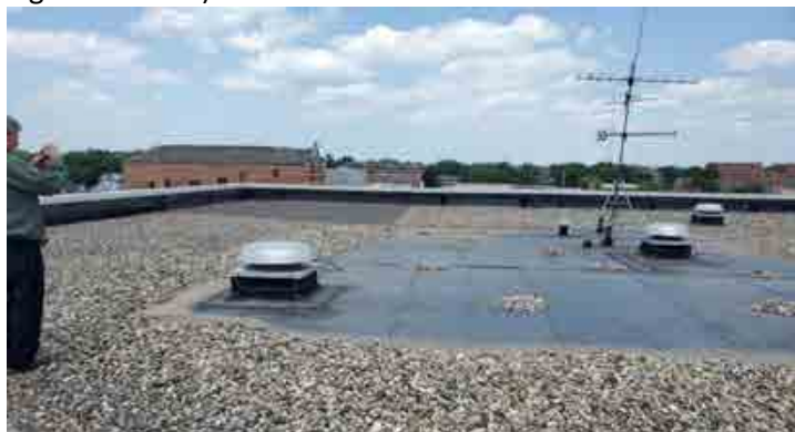
Figure 3. Judicial Center roof: ballasted EPDM.
