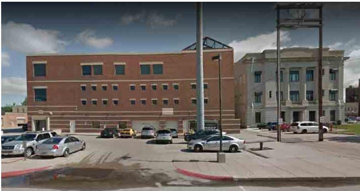
Figure 2. Judicial Center building behind Courthouse (Google Street View)
