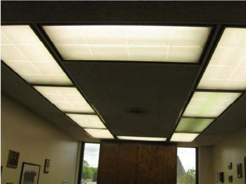
Typical original interior fluorescent light fixtures with discolored lenses
