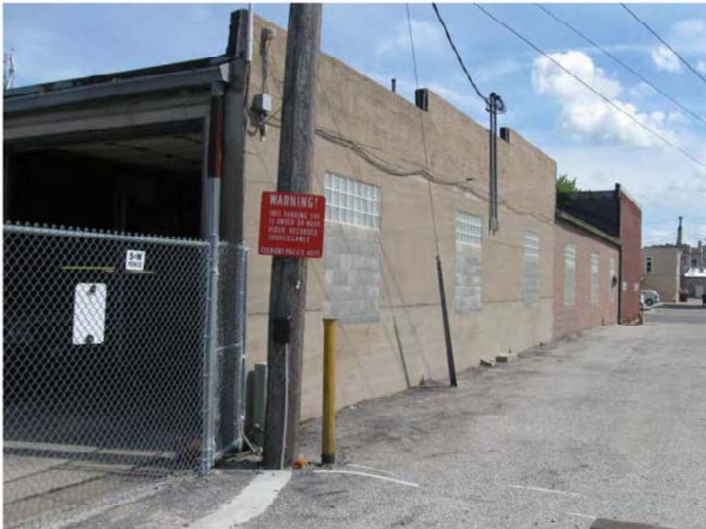
Three sections of garage facility
