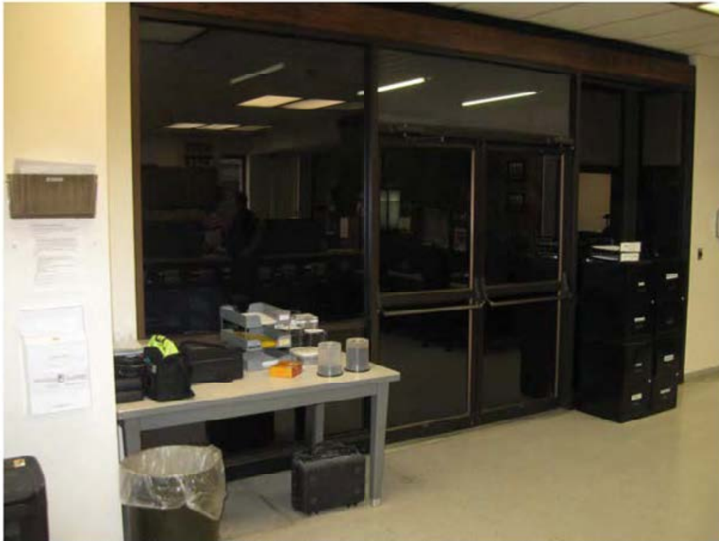
Entrance to Patrol Area with reflective glass (wrong side) and screen mesh above doors
