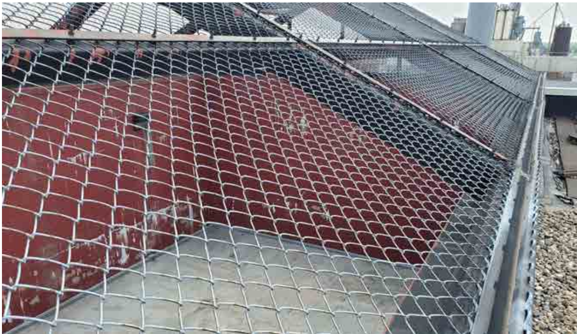
Figure 4. Inmate Exercise Area roof enclosure
