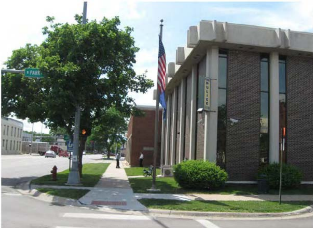
Sign mounted to southeast corner of FPD
