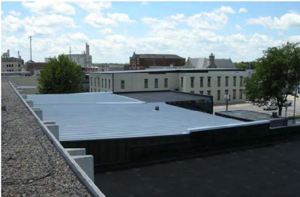
Garage roofs looking south – note maze of roof runoff areas
